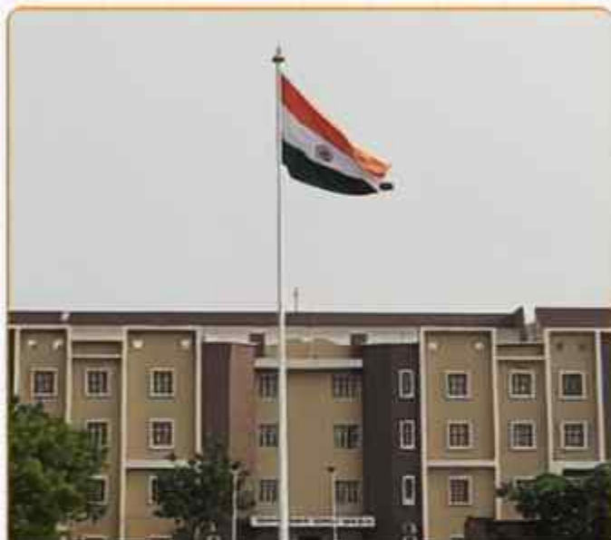
Public Institutional Infrastructure
